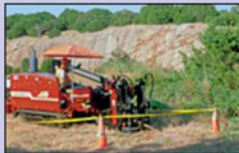
We "know" how to make a successful directional bore shot.
